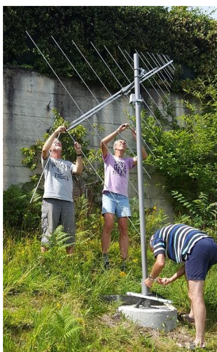
Installation of a logarithmic periodic dipole antenna array (LPDA) at IRSOL.
